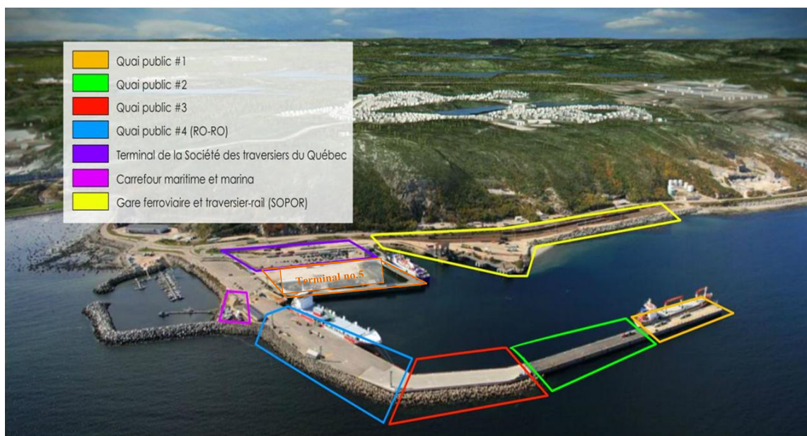
Figure 2. Harbor port Facilities
